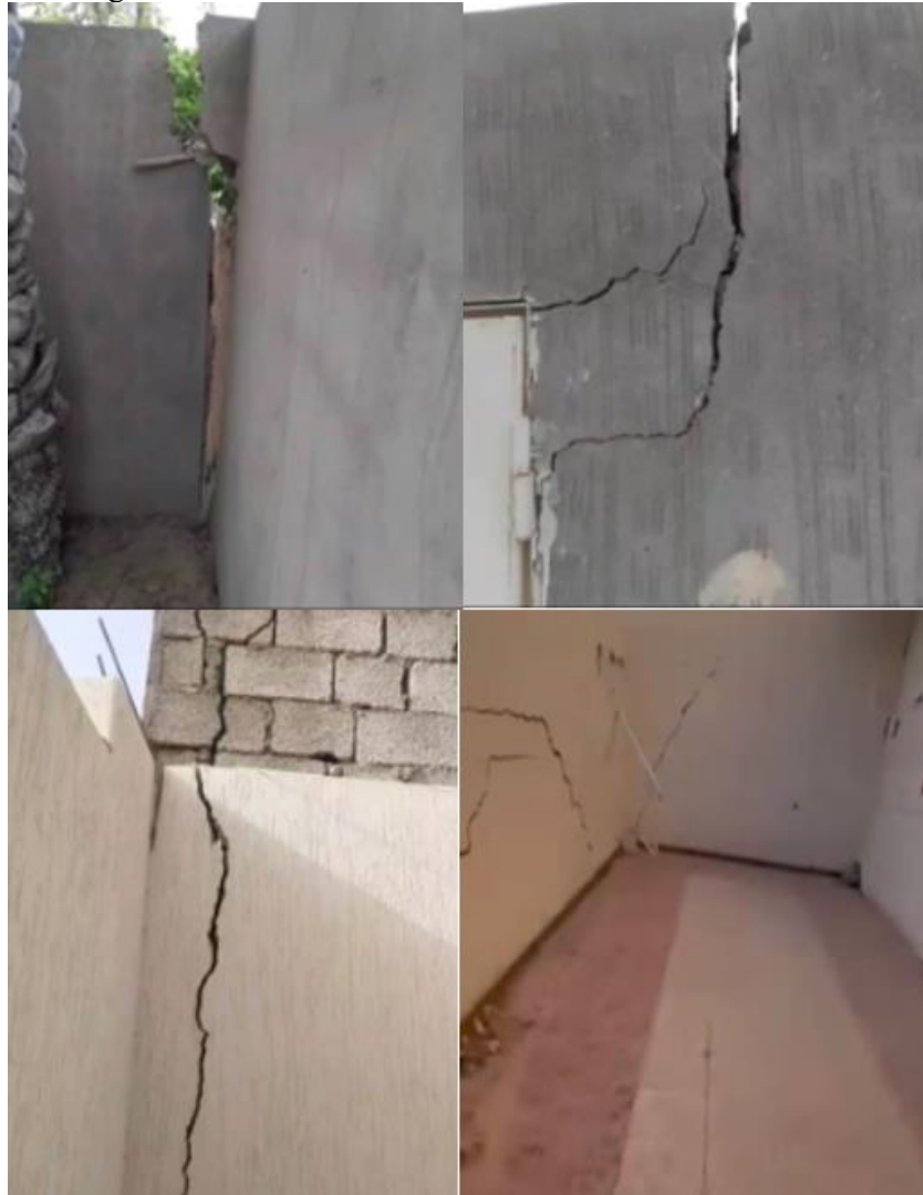
Figure 1. The Impact of Polluted Groundwater on Infrastructure (pictures were taken by the authors)
